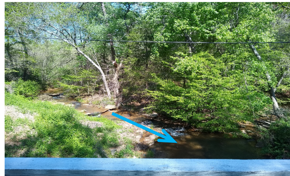
View Looking Upstream from Bridge 336
