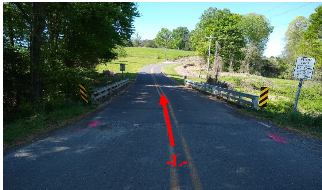
View of Bridge 336 Looking Downstation
