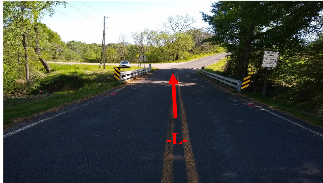
View of Bridge 336 Looking Upstation
